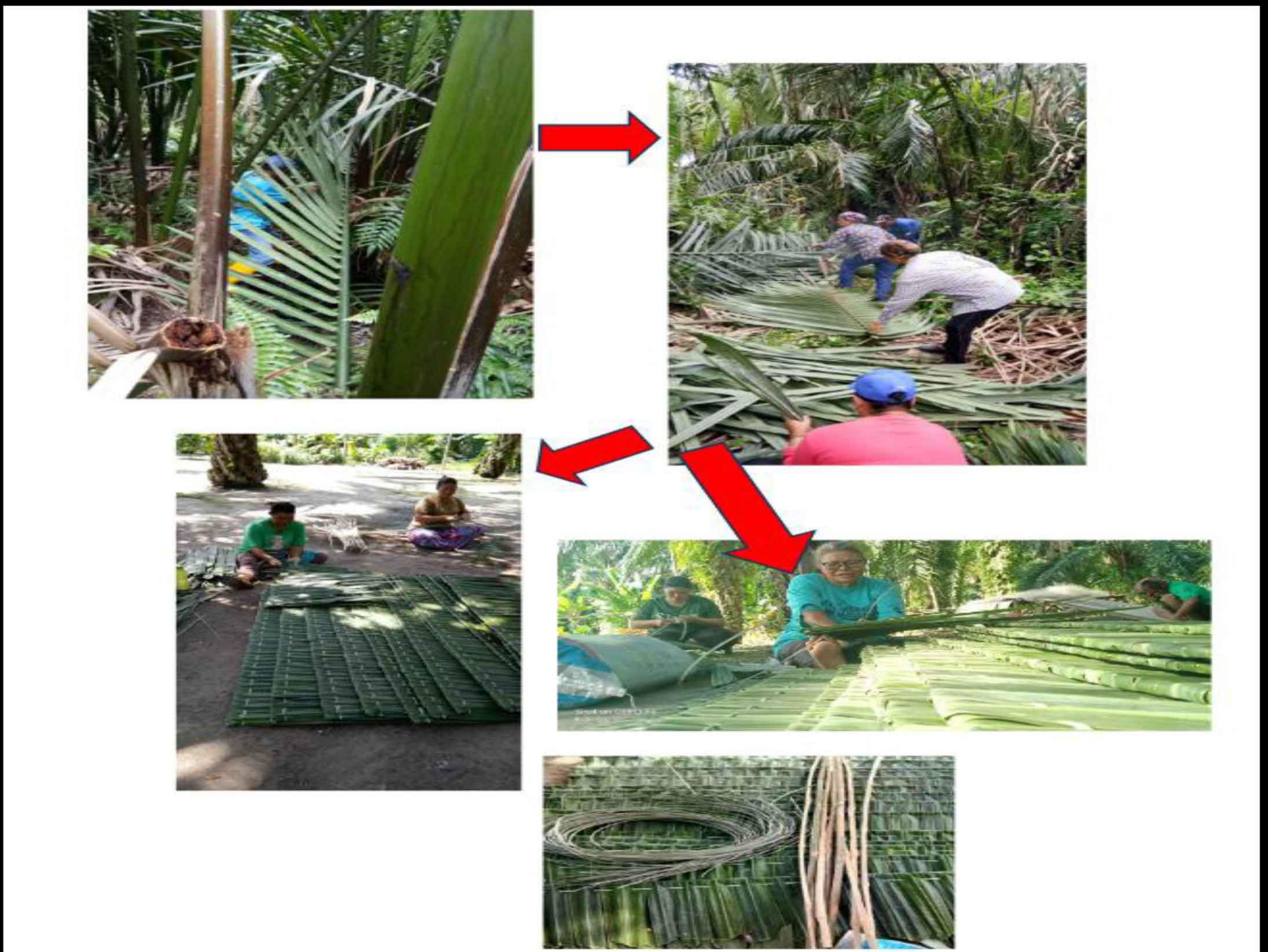
Roofing using nipah leaves made by local people using the traditional technique .
