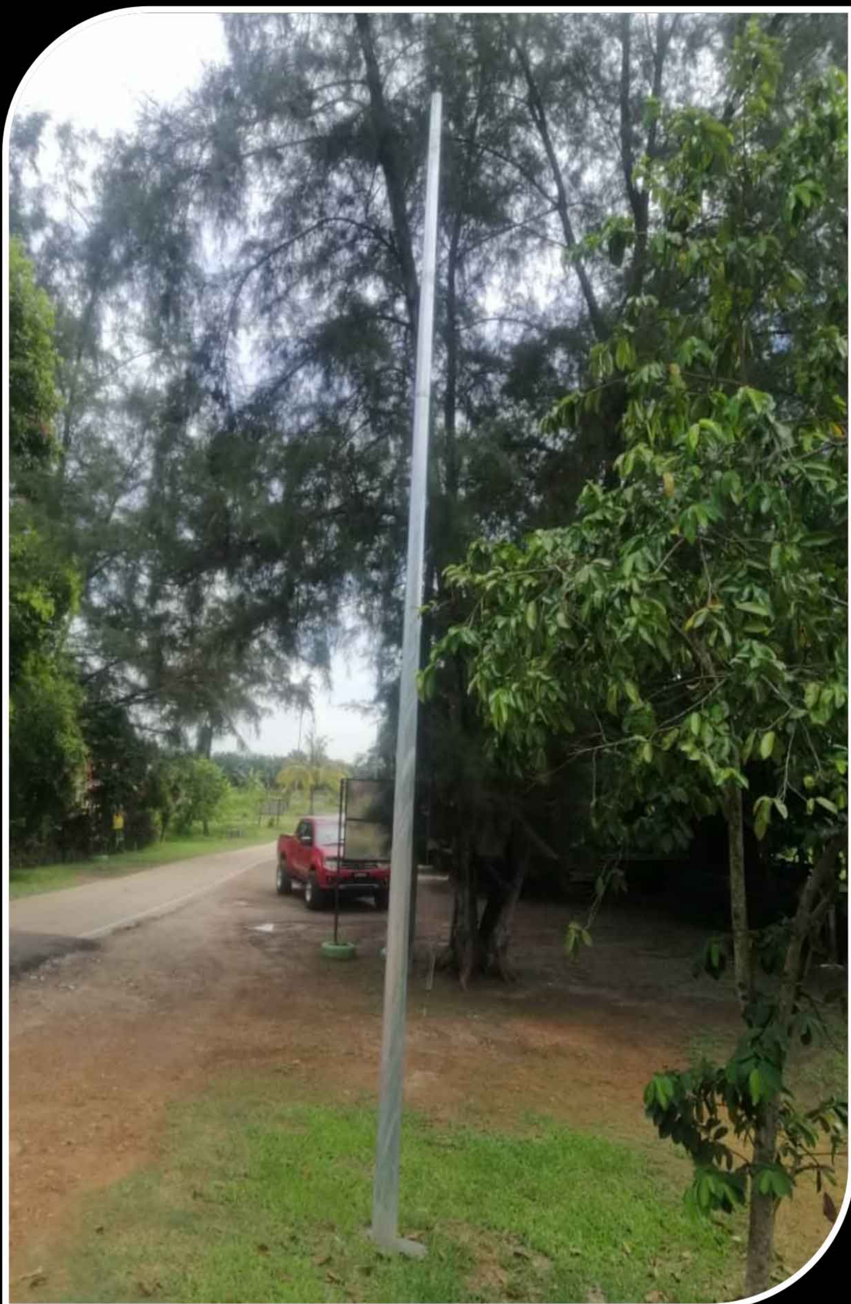
Preliminary work of installing the solar lighting
