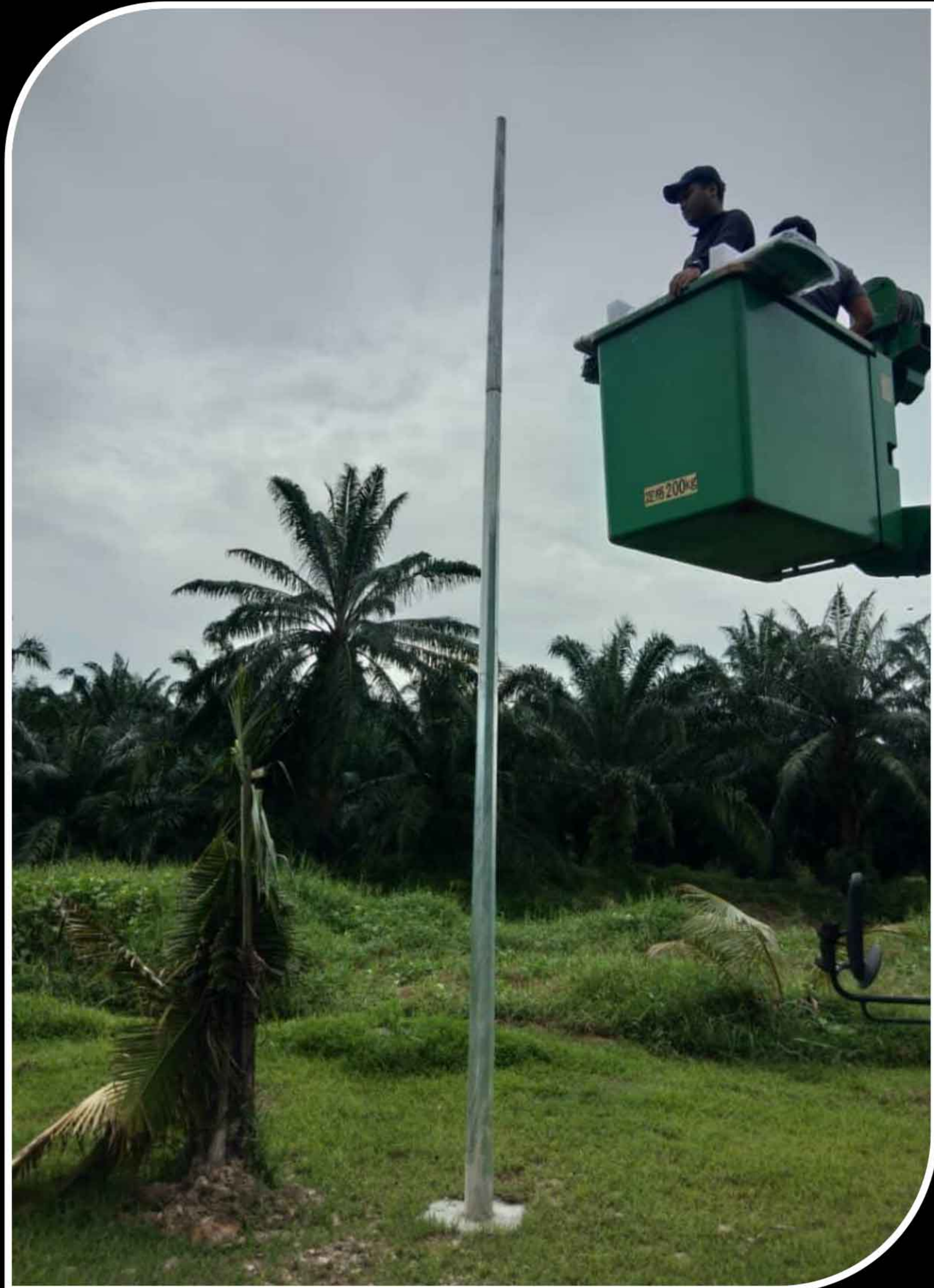
Preliminary work of installing the solar lighting
